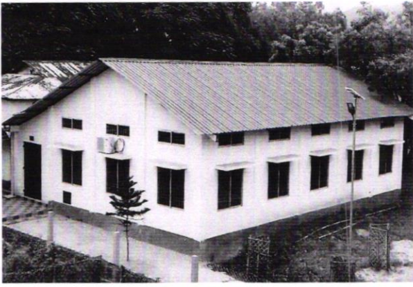
Renovation of Library
