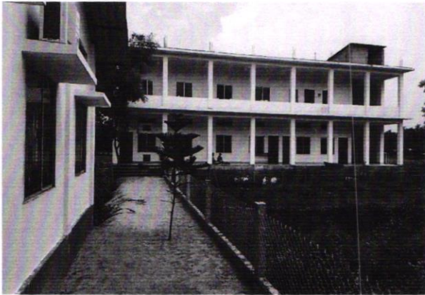
New construction of Classroom & Computer Centre
